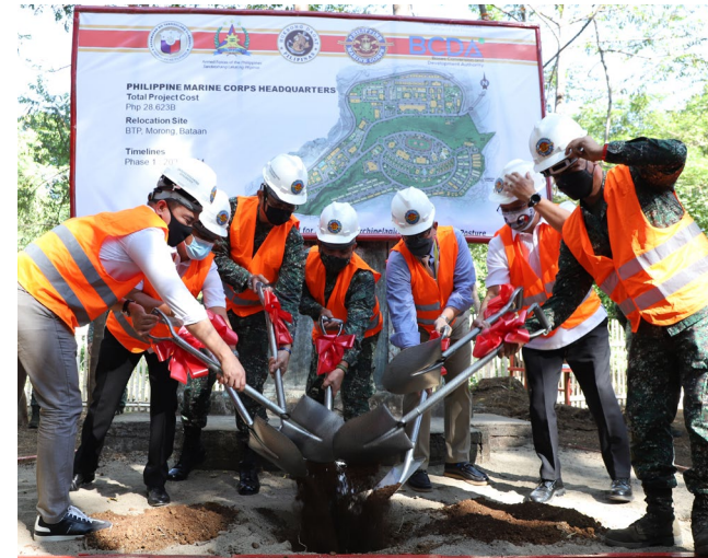
DND, BCDA, and Subic Bay Metropolitan Authority officials at the groundbreaking of the Philippine Marine Corps Headquarters at Bataan Technology Park in Morong.
