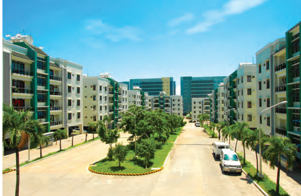
The JUSMAG Officers' Quarters, a Php700-million housing complex, is BCDA's landmark replication project.
