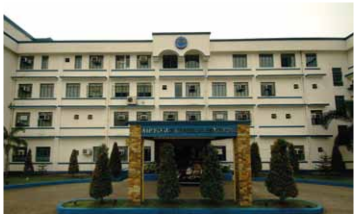
Among replicated projects inside Villamor Air Base is the Philippine Air Force General Hospital.
