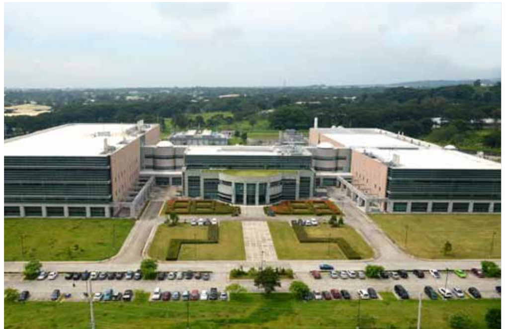
The massive Texas Instruments plant (Photo Credit: Texas Instruments Philippines)
