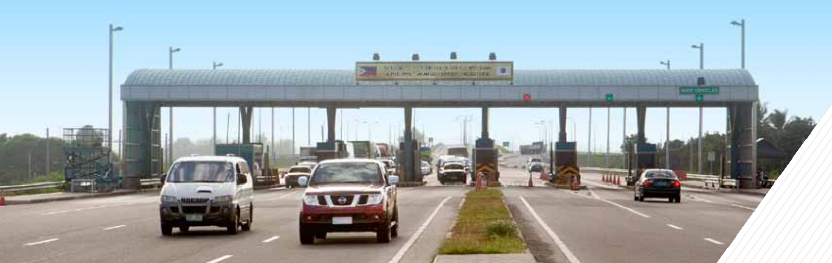
The Clark North Interchange
