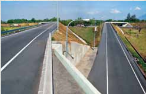
A portion of the Clark North Interchange in Pampanga.
