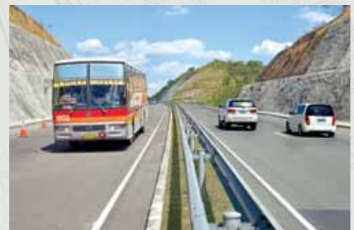
More buses bound for North and Central Luzon provinces take the SCTEX for faster travel.
