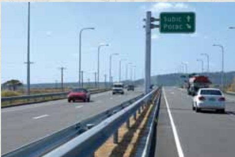
This way to the new Clark South Interchange.
