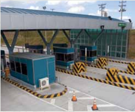
The Porac Toll Plaza
