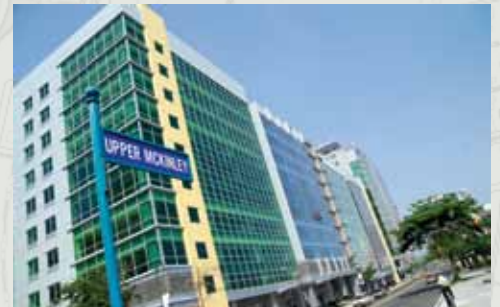
Business Process Outsourcing companies are located at 18 and 20 Upper McKinley Road.
