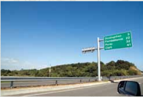
Additional signages are installed along the entire carriageway to guide motorists.
