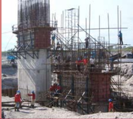
Shown is a reinforced concrete box culvert in Brgy. Dampe, Floridablanca, Pampanga (above) and the installation of rebars of the Pasig-Potrero Bridge at Angeles, Pampanga (below).
