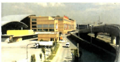
3 August Completion of the Collector Distributor (CD) Road Segment 1–Mabini Ramp and Slope Protection
