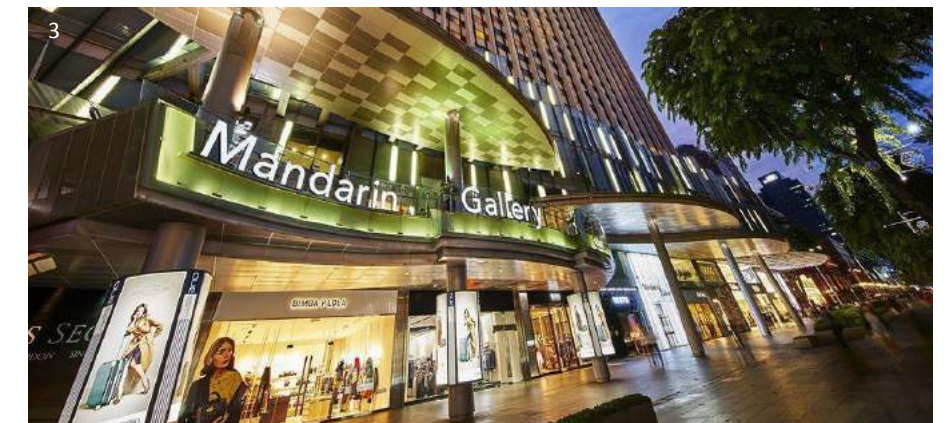
Shopfronts with high level of transparency
