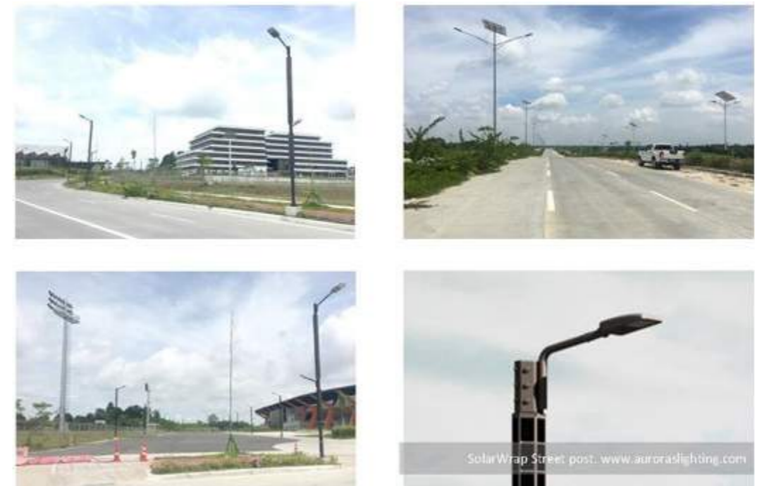
Figure 9.15 Actual Street lights in Phase 1A
