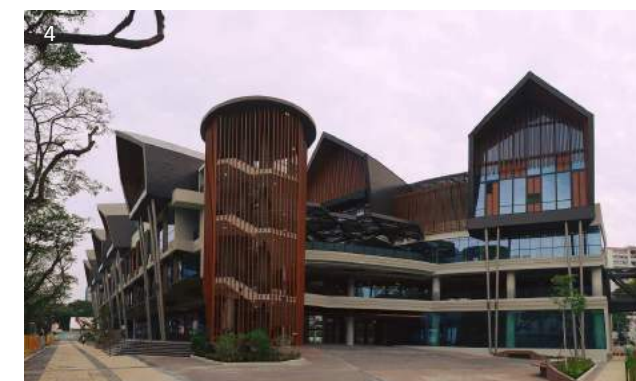
A Building with Vernacular Design Elements
