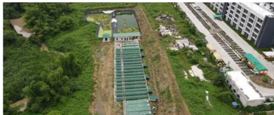
Figure 9.4 Aerial View of Existing STP Source: NGAC Construction Supervision Team
