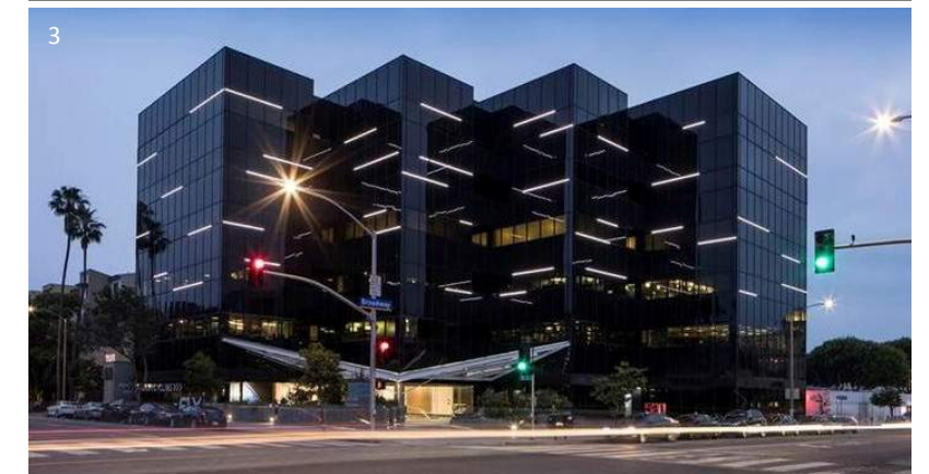
3 North Technopark & Clark Highlands Lighting
