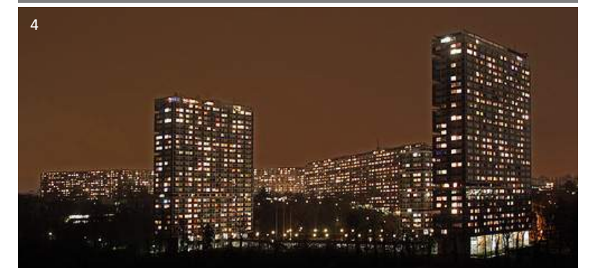
4 North Gate & South Gate Lighting
